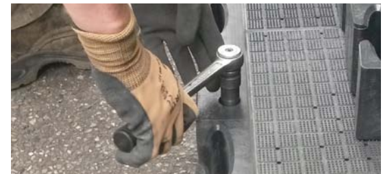
4. To ensure that the rod is correctly anchored, it should be rotated while being inserted into the hole (full of resin) so that the thread is packed completely with resin
