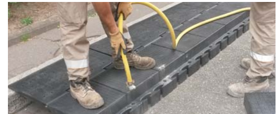
2. Cleaning the holes.
