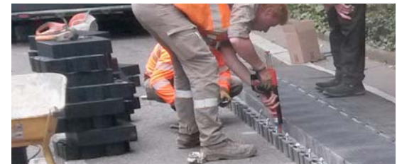
3. Filling with resin
